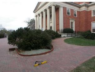
Figure 4 - 7.6% Cross Slope on Approach Walk
