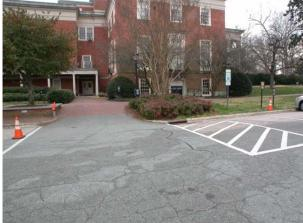
Figure 2 – Inaccessible Eastern Curb Ramp
